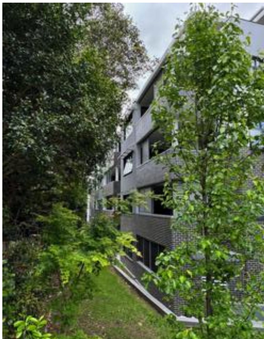
9. View of No. 9-21 Lorne Ave
