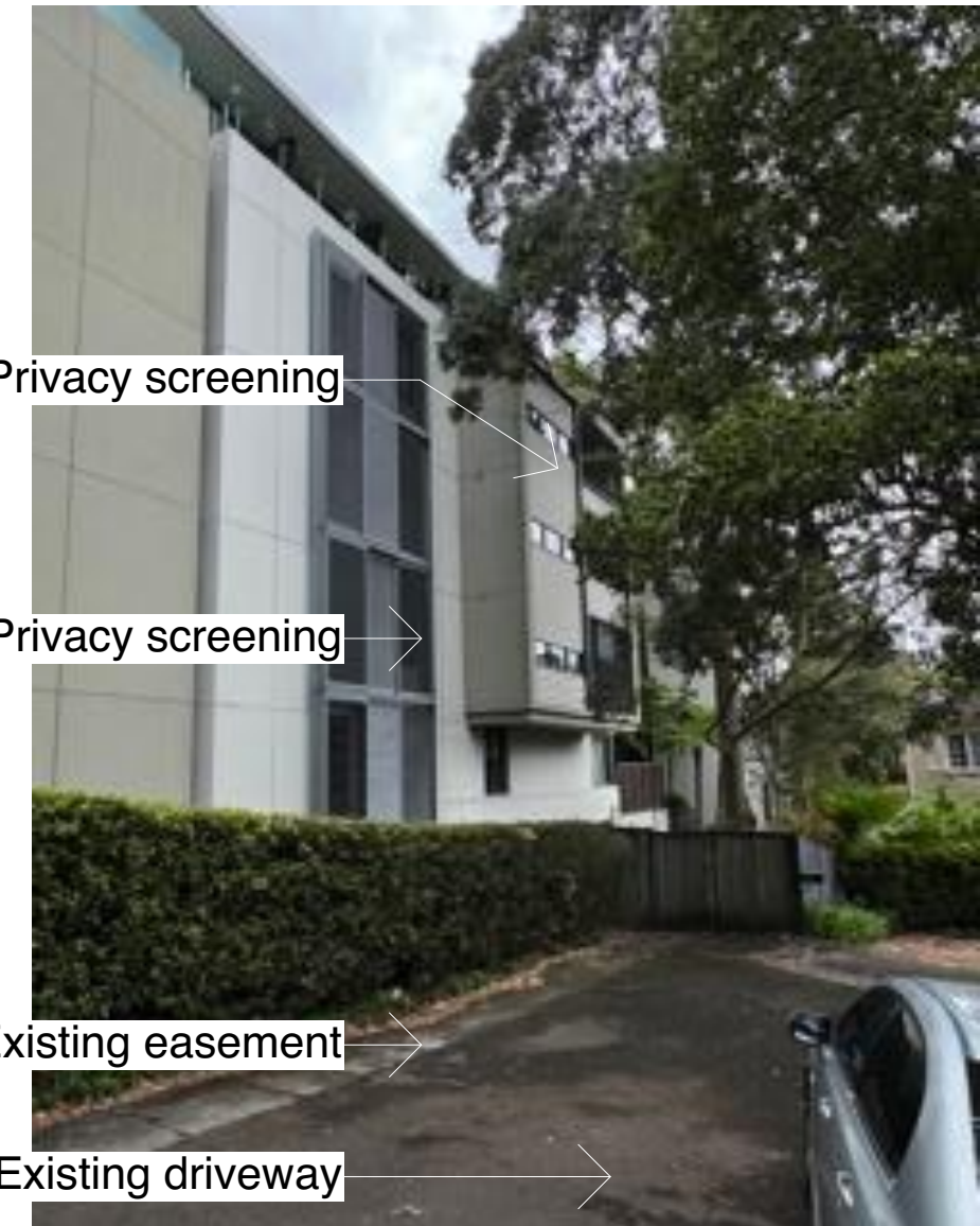
6. View of No. 25A, 27 and 29 Lorne Ave
