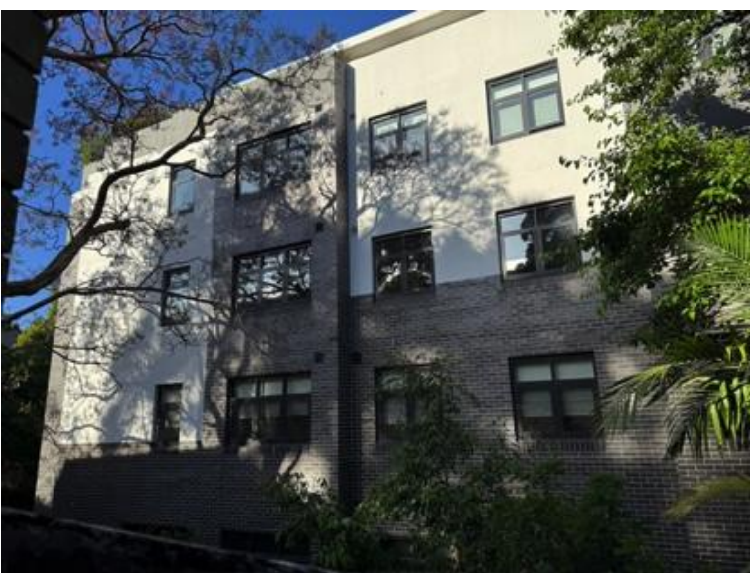
11. View of No. 9-21 Lorne Ave
