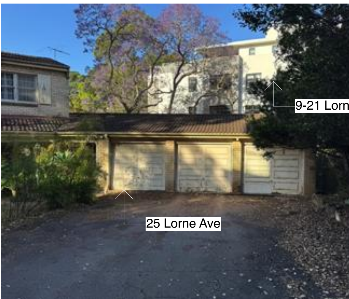
7. View of No. 25 Lorne Ave
