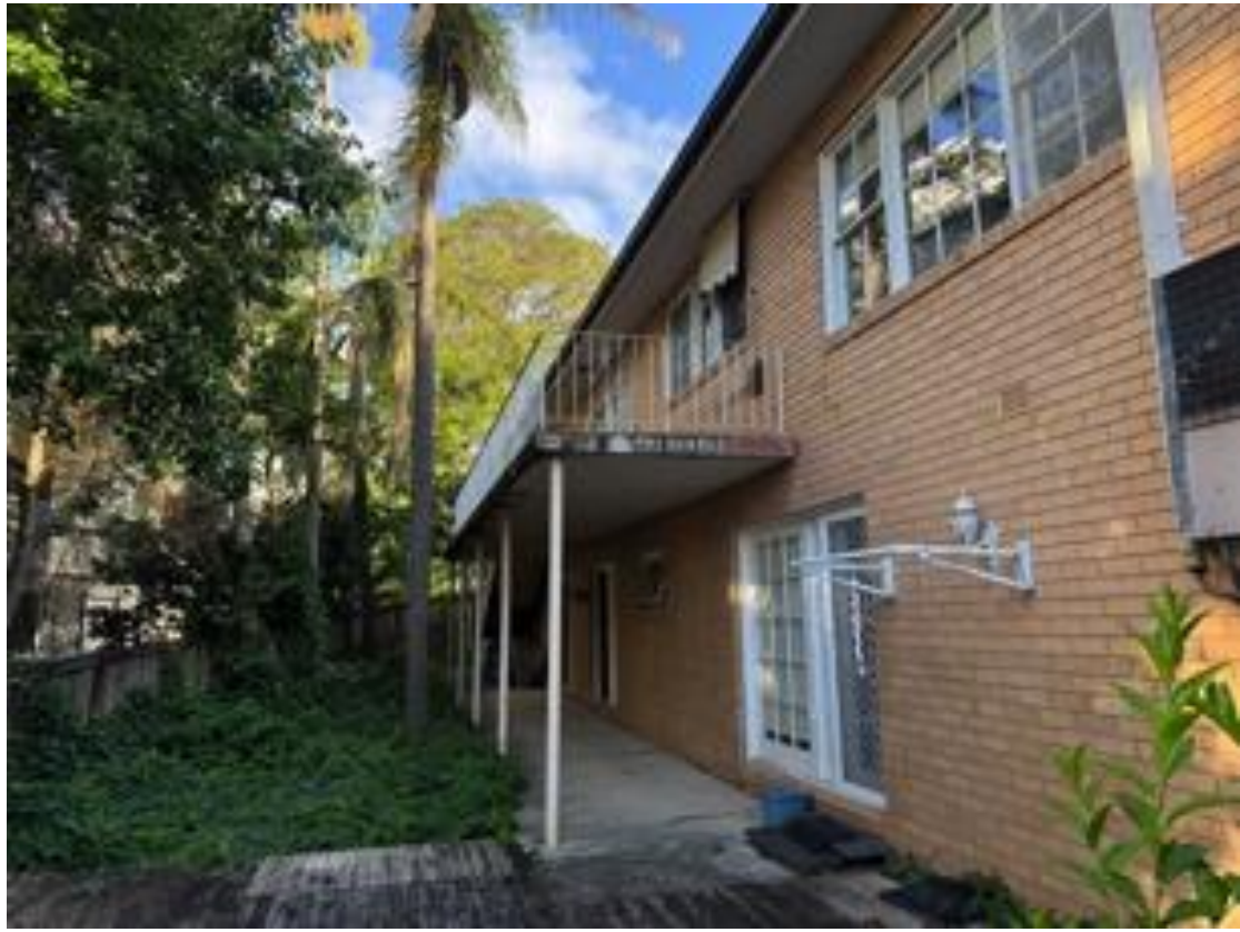
10. View of No. 23 Lorne Ave
